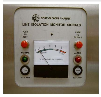
INFORMATION: Line isolation monitor alarms play an important role in patient and user safety. Whenever these devices go into alarm, there is an unsafe electrical condition in some electrical piece of equipment.
